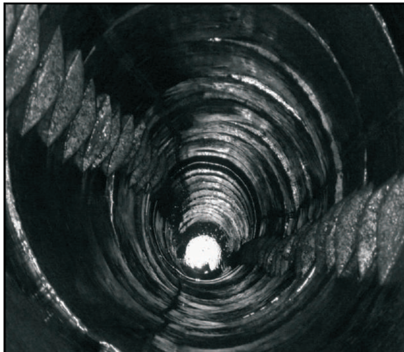
Figure 2: Well water vividly polluted with oil at one of the fuel stations.
