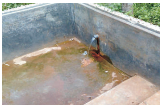
Figure 4: A protected spring with adequate drainage of waste water
