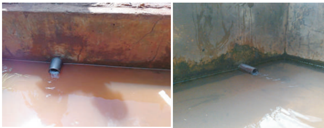
Figures 2 and 3: Two protected springs with water stagnated in the collection chamber.
