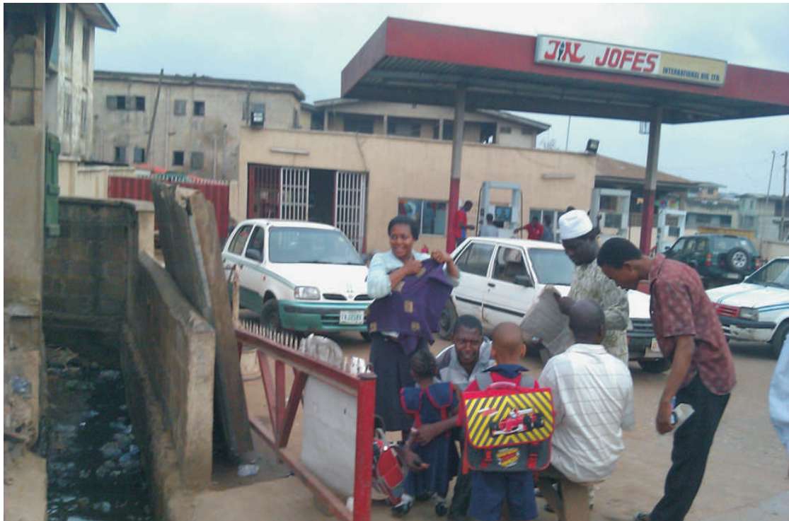
Plate1: JIN JOFES petrol station with less than 7 meters from a residential building Source: Authors' Field Survey, 2012
